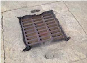
These drains also called catch basins are used to collect the stormwater, in our case normally rain water, and direct it into a system of underground pipes that flow to the west to an unnamed tributary channel of Snow Creek.
